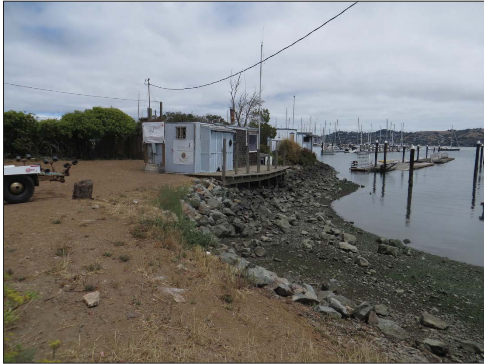
Above: Cass Marina structures and shoreline.
